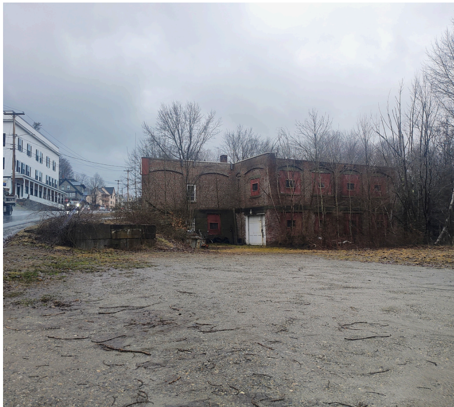
Existing parcel condition; old gas station and repair shop currently used for storage.
