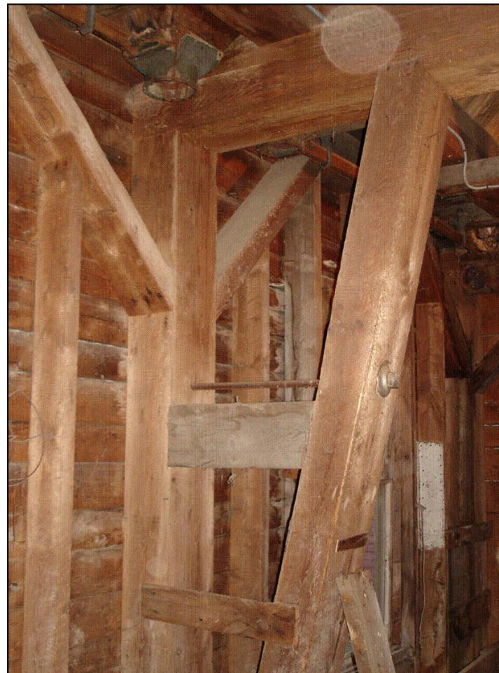
Post and beam framing on first floor
