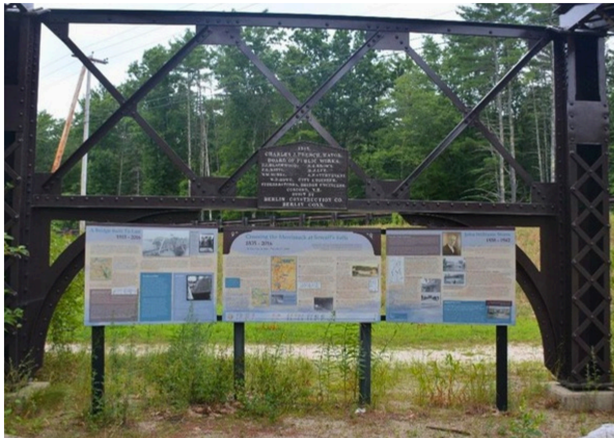
Educational panel highlighting the historical significance of a bridge along a rail trail in Concord, NH
