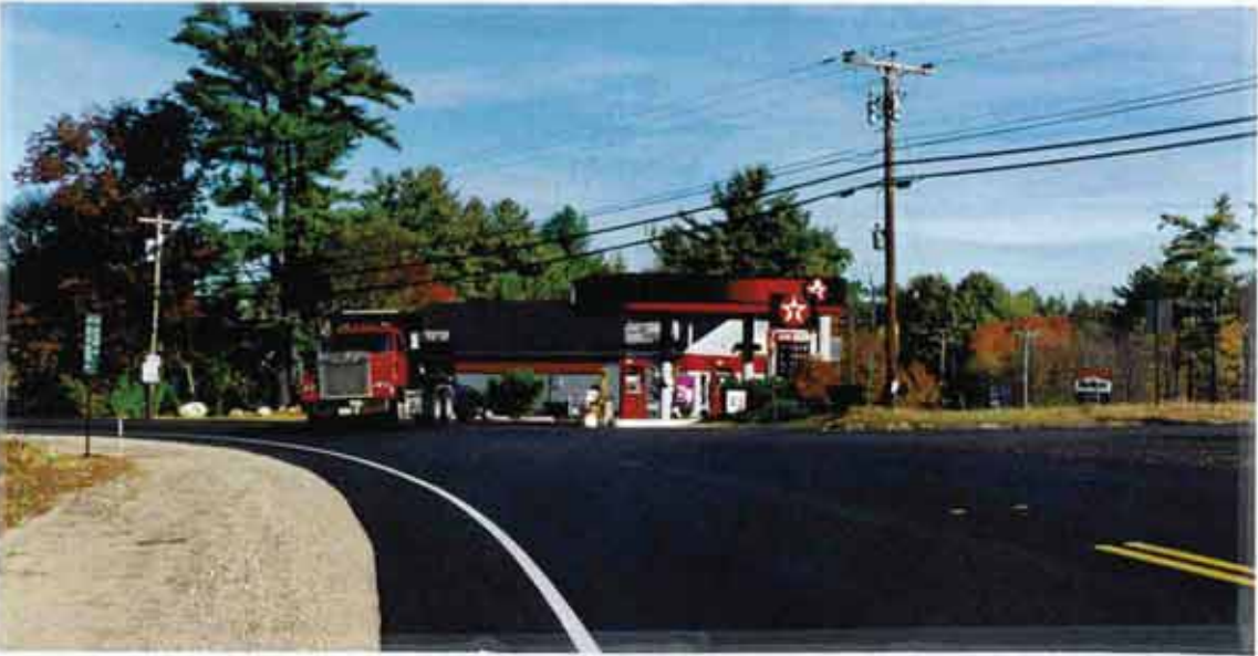
Highway Access To Proposed Public Works Facility
