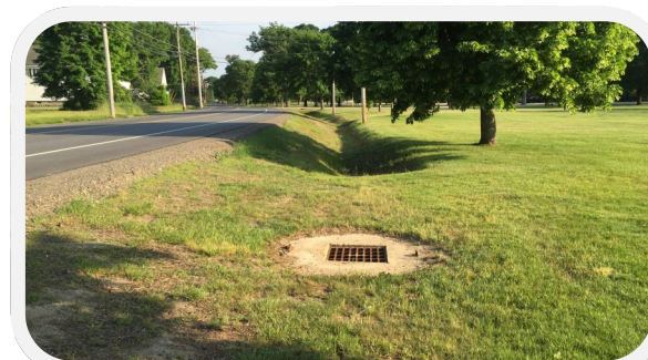
Installing a porous multi-use path in the current swale location could allow for water to flow to the path and infiltrate into the ground.
