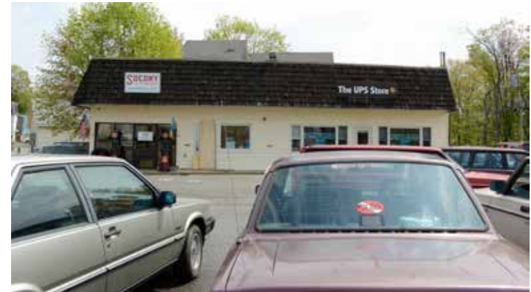
Existing facade of the Volvo building
