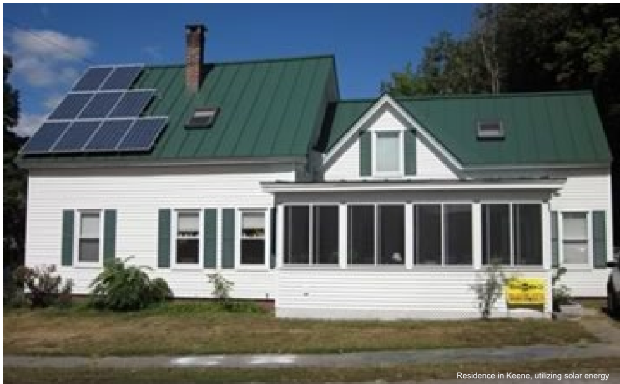
Residence in Keene, utilizing solar energy
